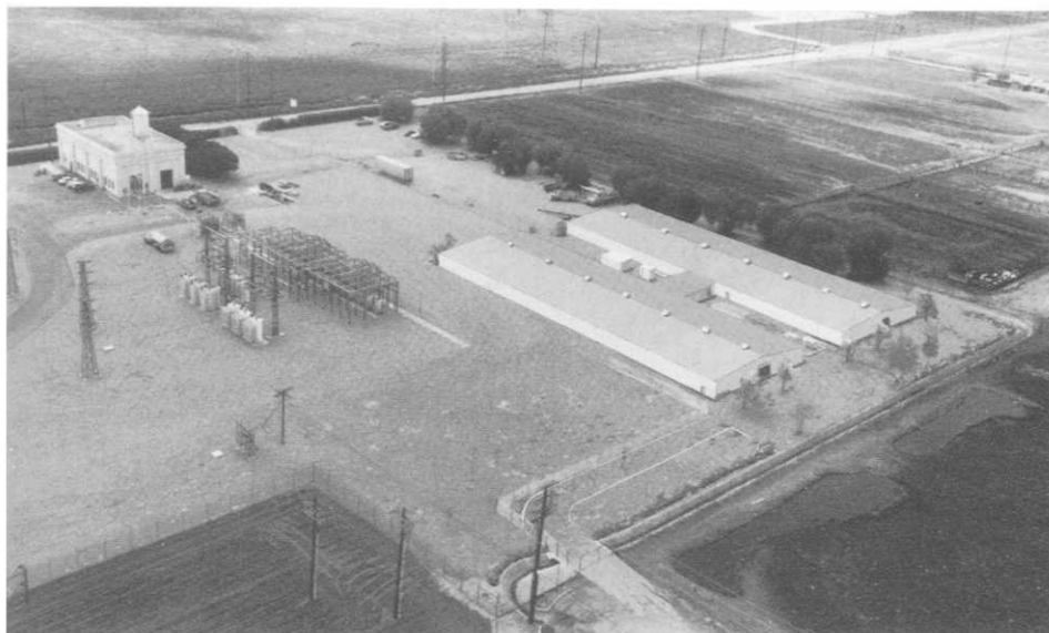
Fig. 3. Aerial view of Chino 10 MW lead/acid battery energy storage project.
